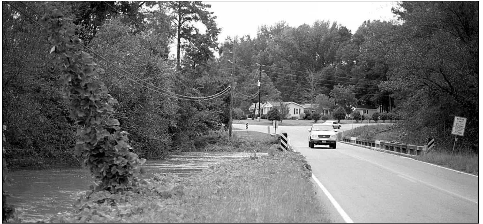
This bridge over Swift Creek at Barber Mill Road in south Cleveland barely avoided meeting its demise in the aftermath of Hurricane Floyd on the night of Sept. 15. By Thursday morning, the waters had risen to within three feet of the bottom of the bridge.
